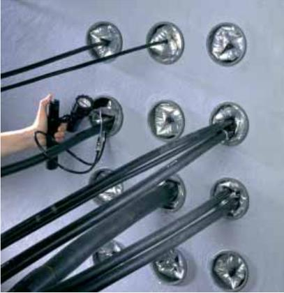
TDUX is a unique inflatable wraparound duct sealing system for permanently sealing telephone cable ducts in order to prevent the leakage of water from the duct into exchange vaults or manholes. It has been developed for use with plastic, concrete or steel ducting wall-feedthrough systems. It can be used with polyethylene or lead-jacketed cables.
