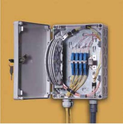
The FIST-SB2-8 is a small wall-mountable customer fiber termination box, offering the functions of splicing fiber-to-fiber, splicing fiber-to-pigtail and connector patching.
