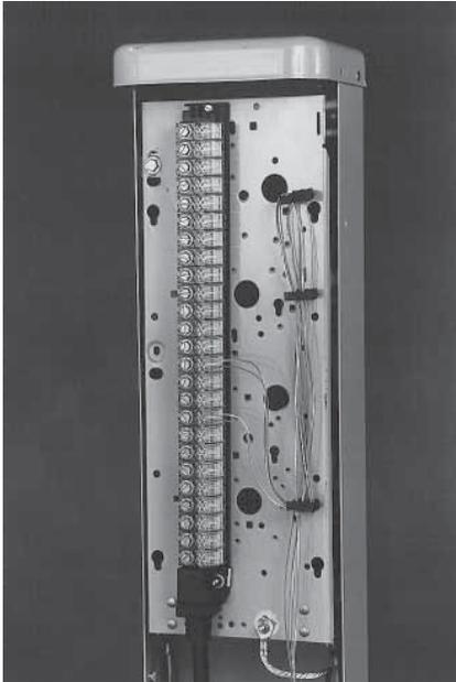
The DTerminator 2 PTB pedestal-mounted terminal system utilizes Tyco Electronics GelGuard technology for environmental protection of the wire connections. The PTB block offers enhanced characteristics, with a versatile mounting system suitable for attachment to any pedestal faceplate. The
