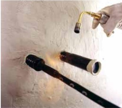
The EPAF wall feedthrough system consists of a heat-shrinkable tube on a steel spring.
